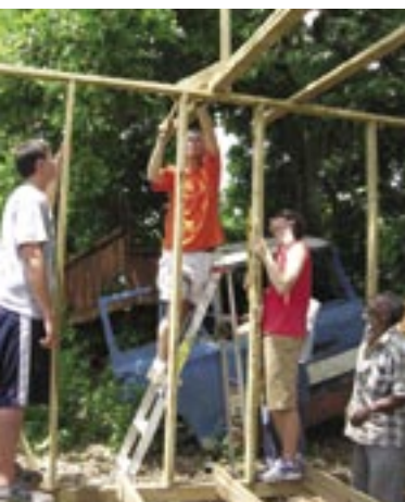
Fr. Jim, in orange shirt, and others work on the frame.
