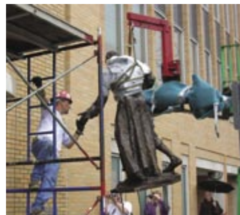
St. Francis being hoisted up.
