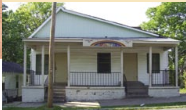
The future home of the Christian Service Technology Learning Center.
